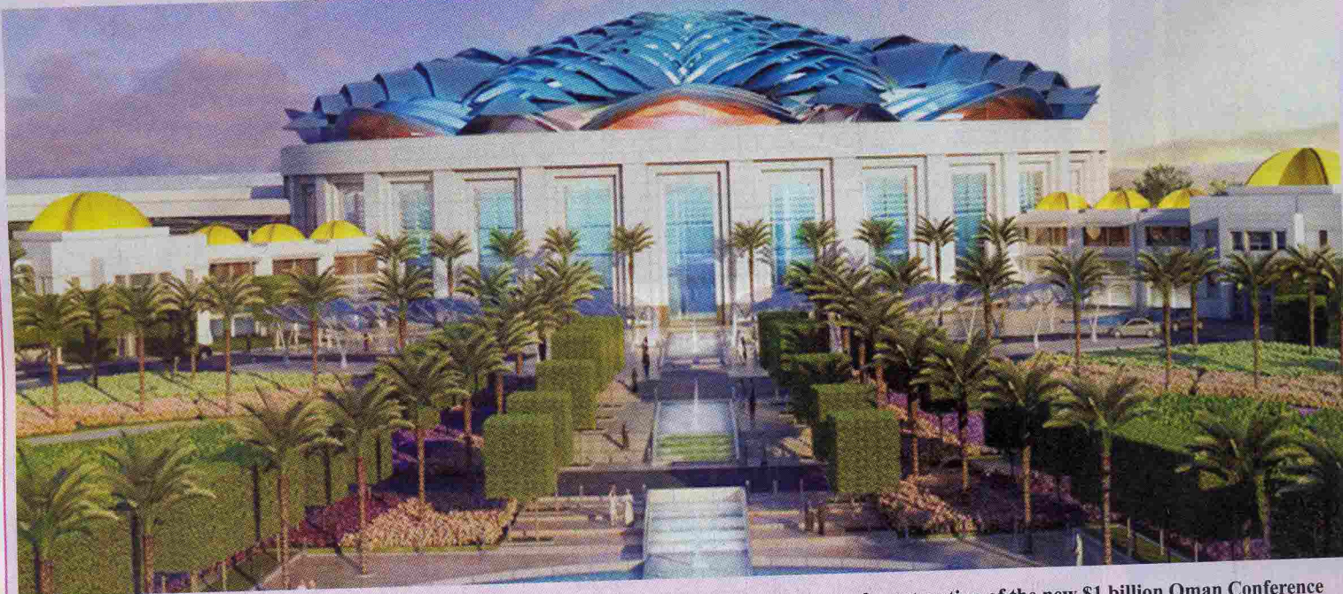
BOOST TO TOURISM: Business tourism is poised for growth following the commencement of construction of the new $1 billion Oman Conference and Exhibition Centre in Muscat. The facility will transform Oman into a key destination for major business events in the region. ■ Details, P4
